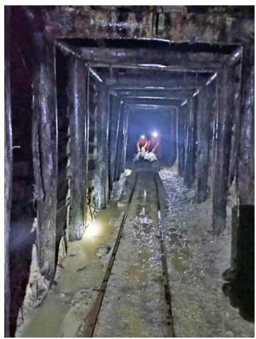
Figure 1: Photograph of underground rehabilitation work currently being done at the Bethania silver mine, Peru. Here, workers are transporting support timbers though a newly-reconditioned section of the mine.
